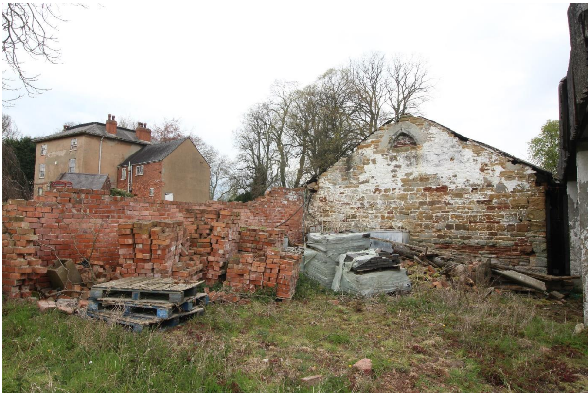
Figure 95 South elevation of Building 4, looking north-west
