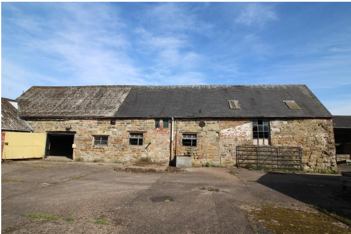
Figure 43 West elevation of Building 5, looking east
