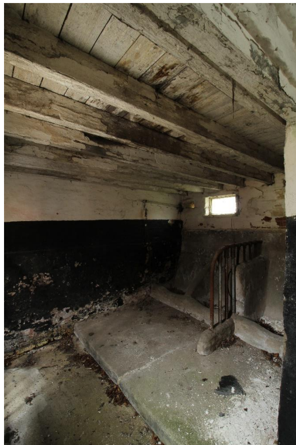
Figure 89 Interior of the northern bay of Building 9, looking south-west
