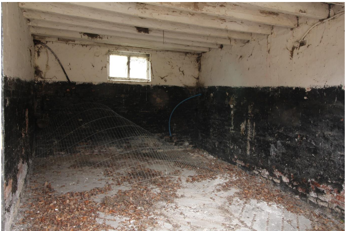
Figure 93 Ground floor of the north bay of Building 11, looking west
