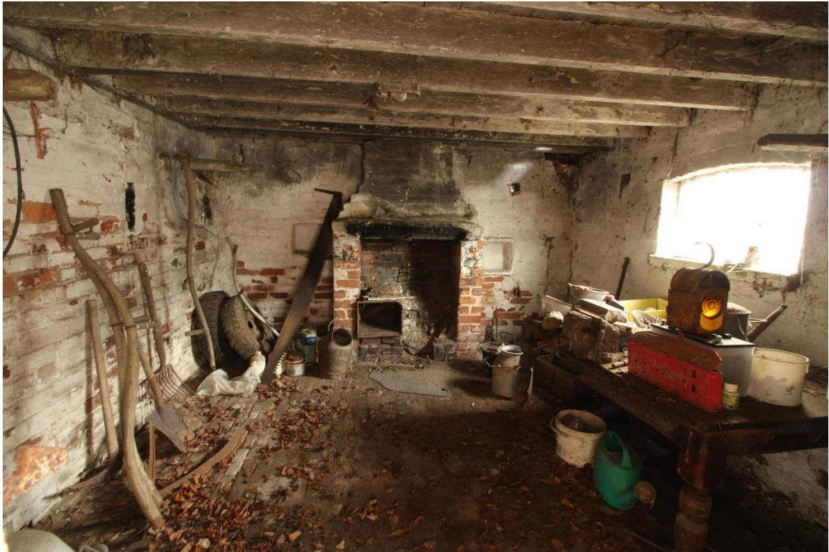
Figure 90 Interior of the south bay of Building 9, looking north
