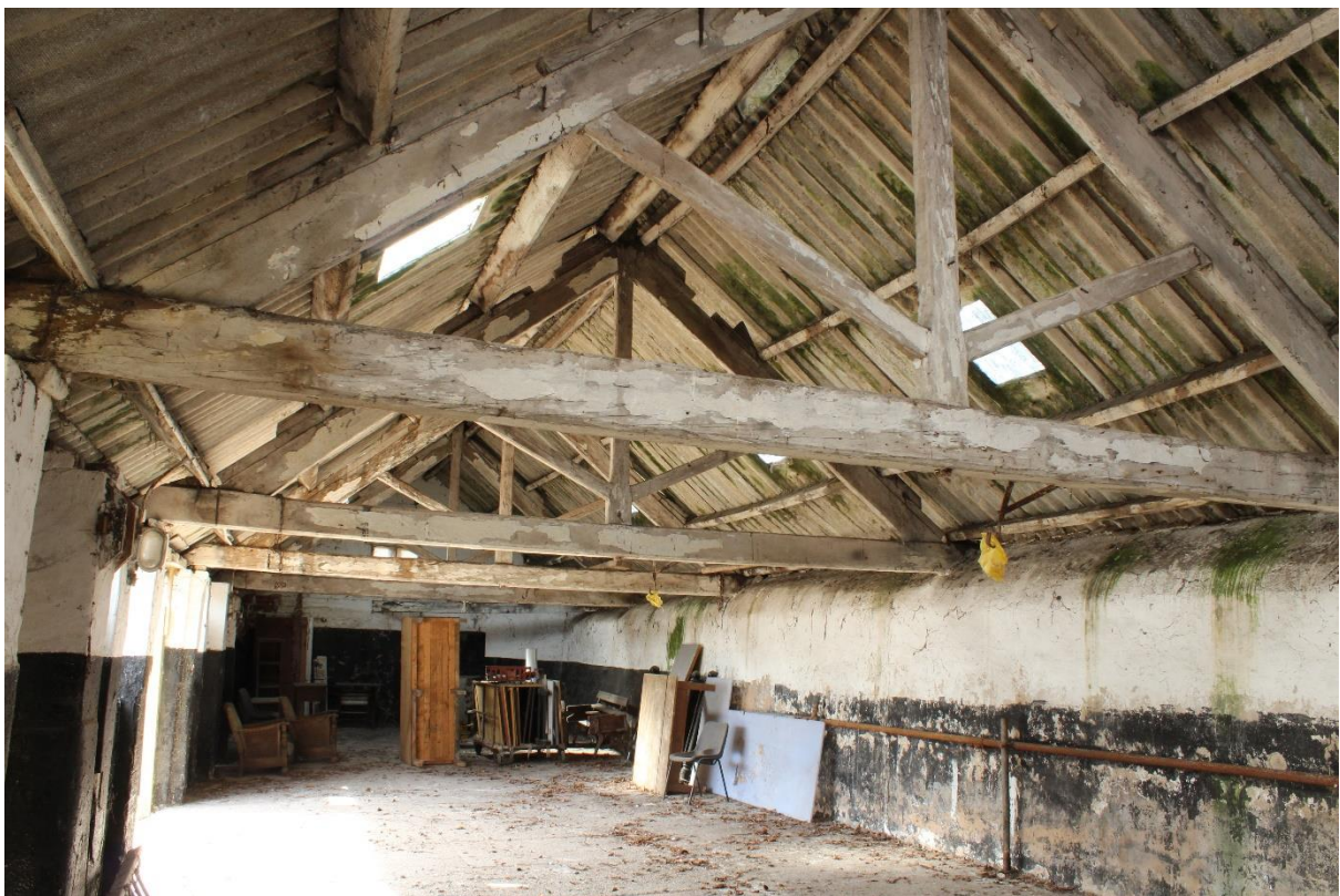
Figure 85 Interior of Building 8, looking west
