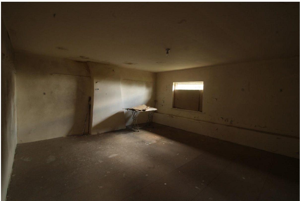
Figure 77 Farmhouse second floor south-eastern bedroom, looking south-east
