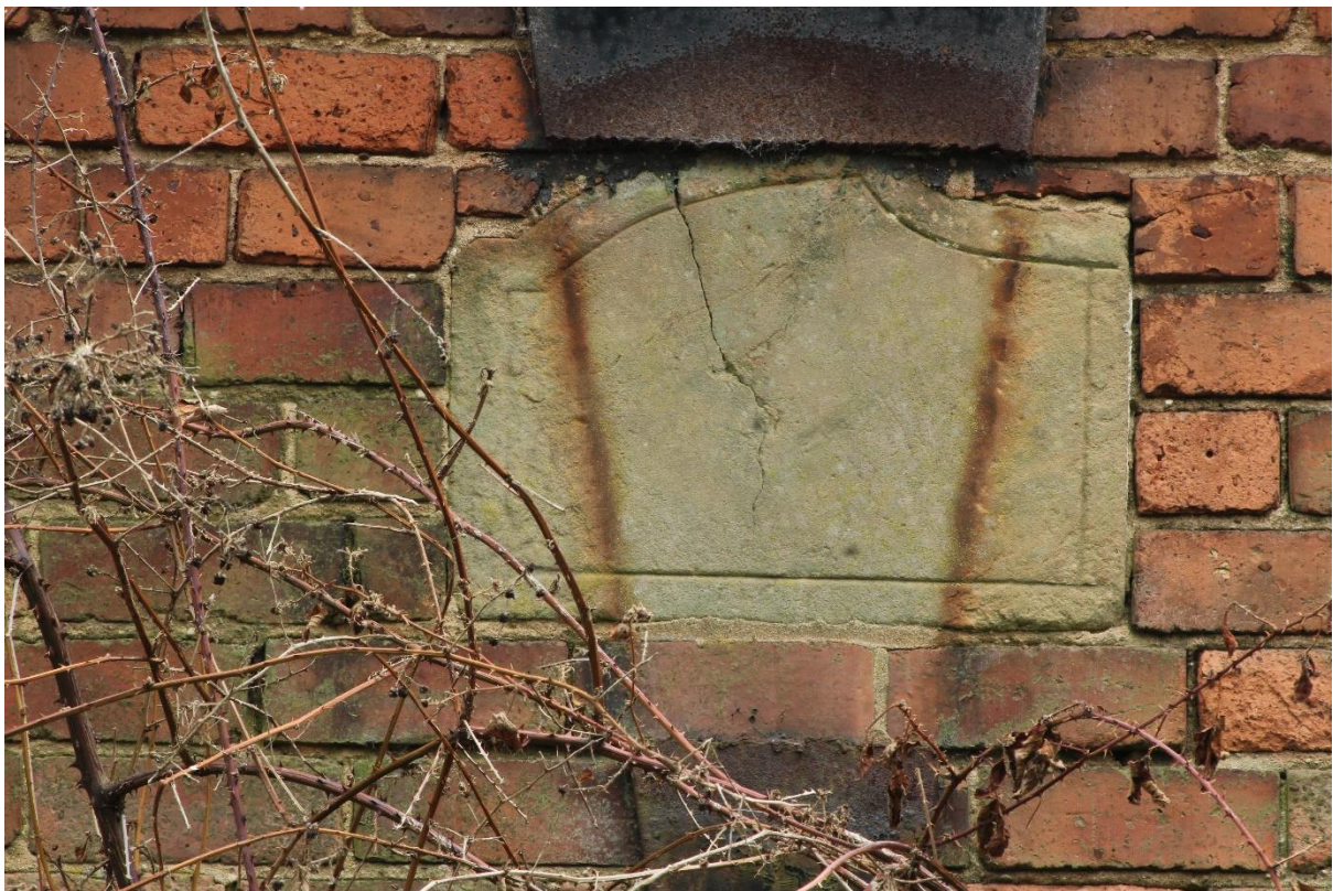
Figure 27 Rebated stone reused in Building 9 (Ex Situ Feature Number 003), looking east
