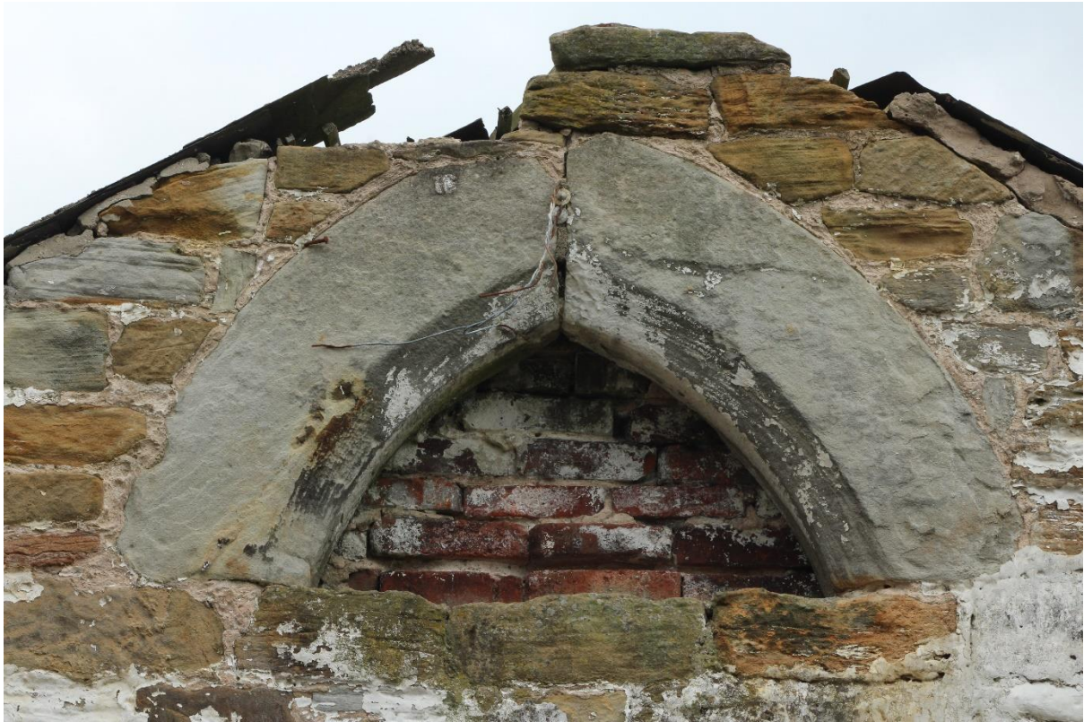
Figure 30 Chamfered door crown reused in the south gable of Building 4 (Ex Situ Feature Number 006), looking north
