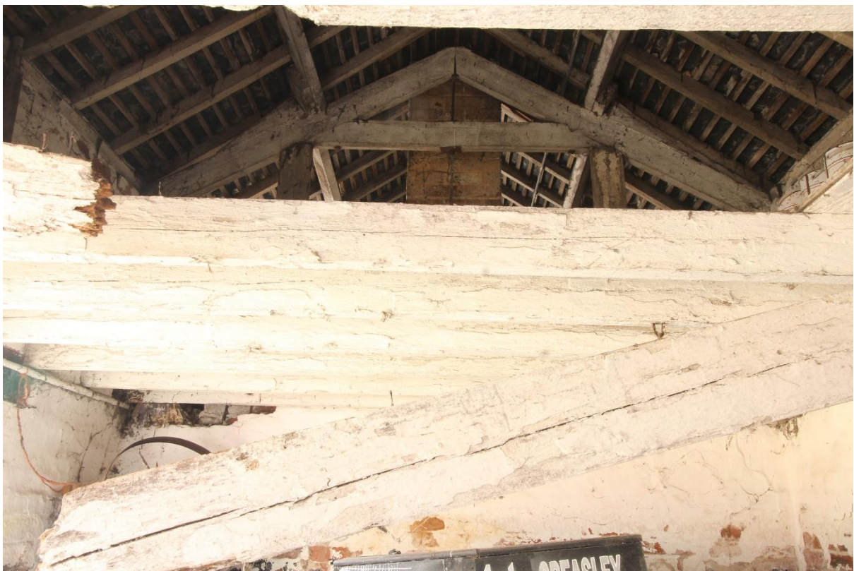
Figure 91 Queen post roof of Building 9, looking south
