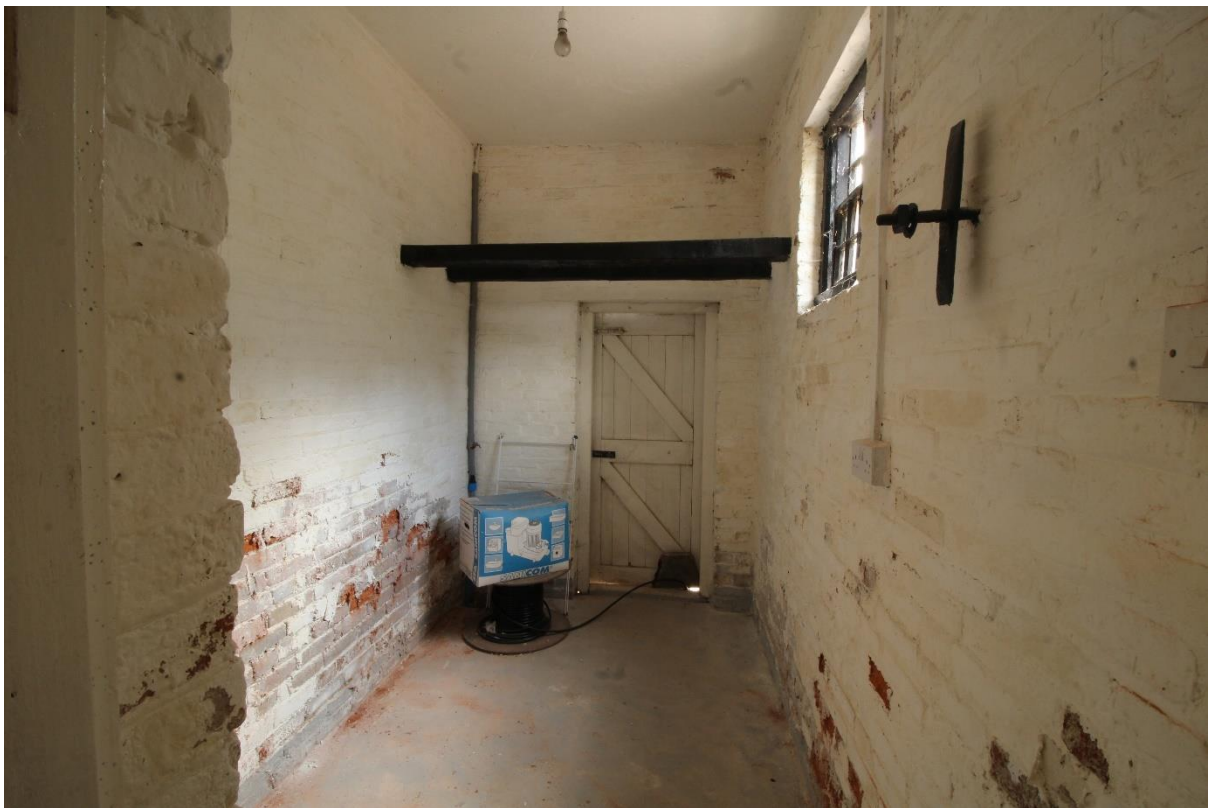
Figure 69 Possible former dairy in the farmhouse east extension, looking east
