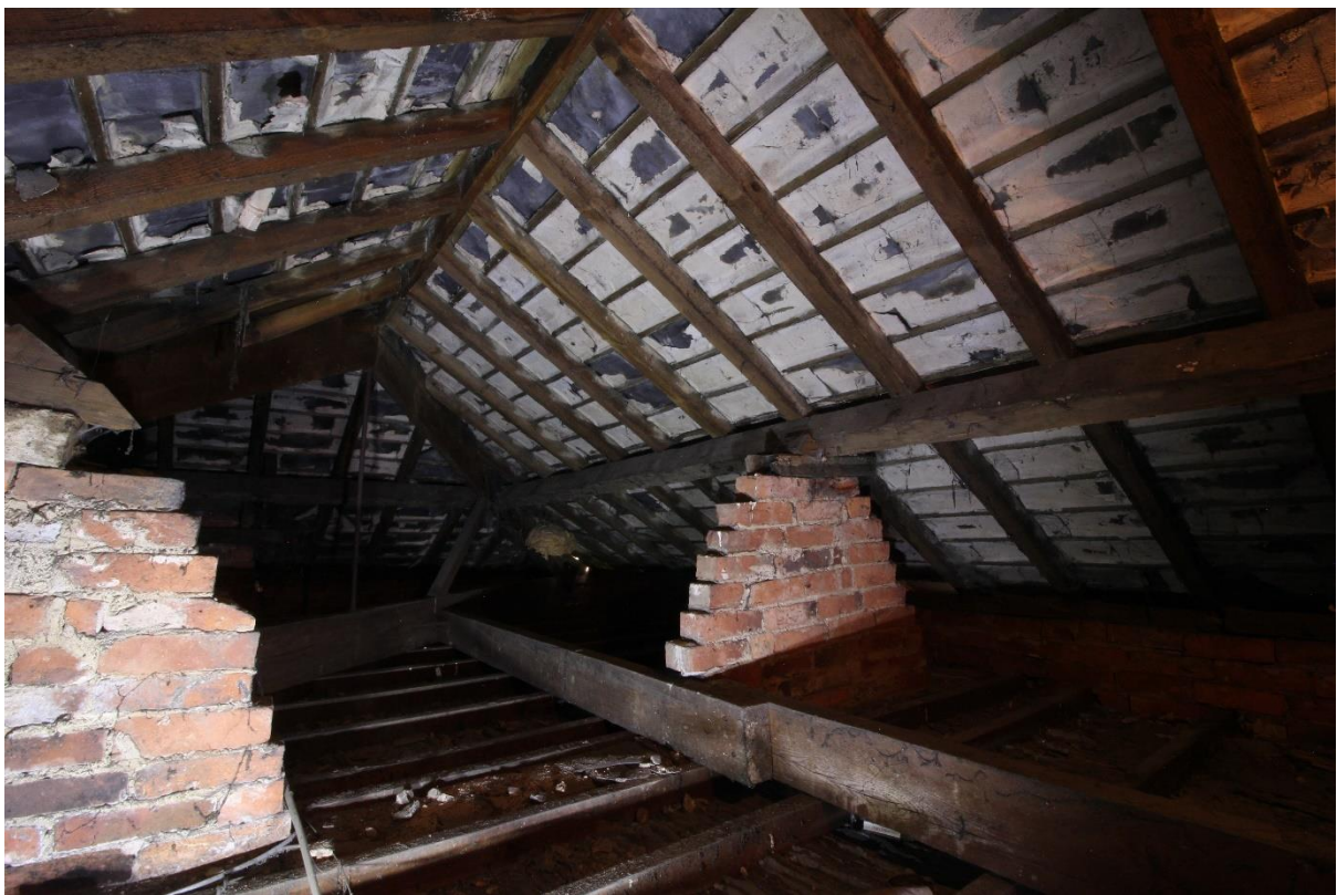
Figure 79 Roof structure of the farmhouse, looking west
