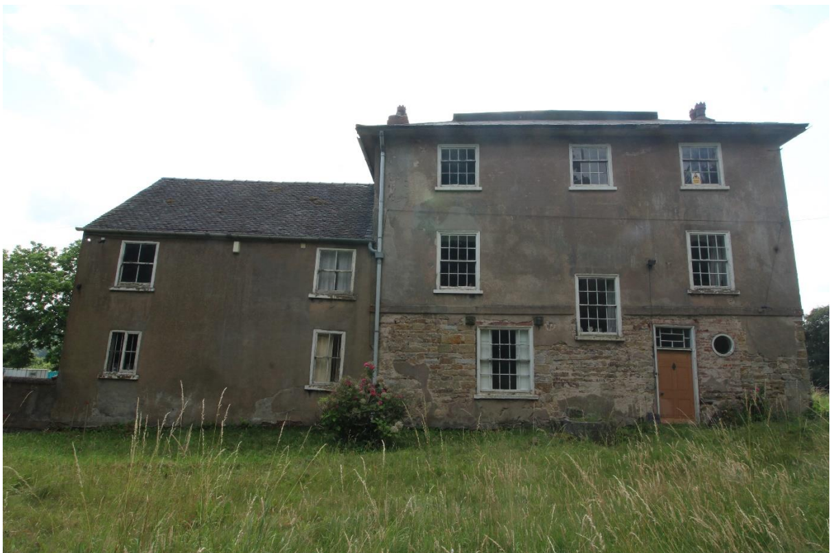
Figure 51 North elevation of the farmhouse, looking south
