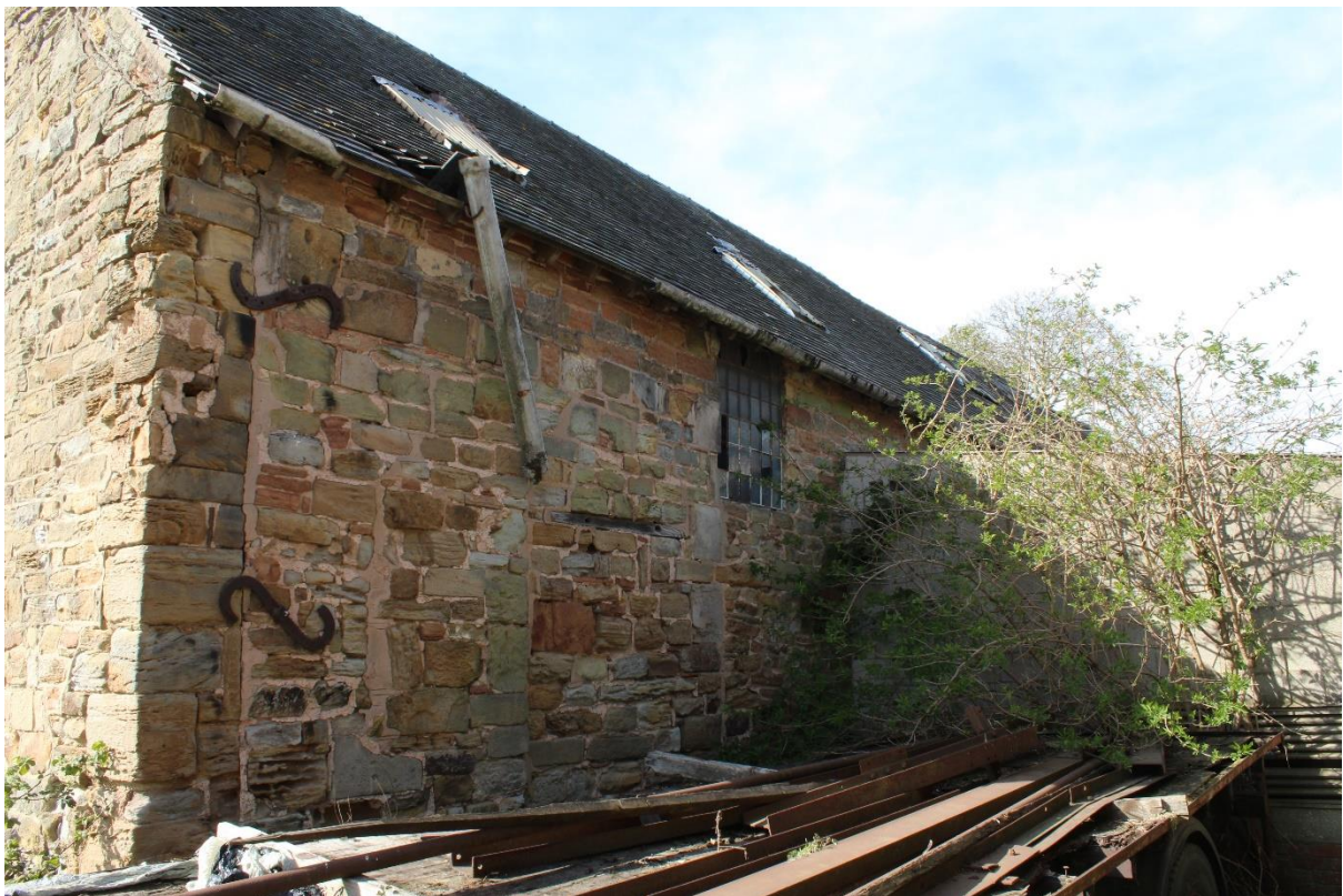
Figure 49 South end of the east elevation of Building 5, looking north-west
