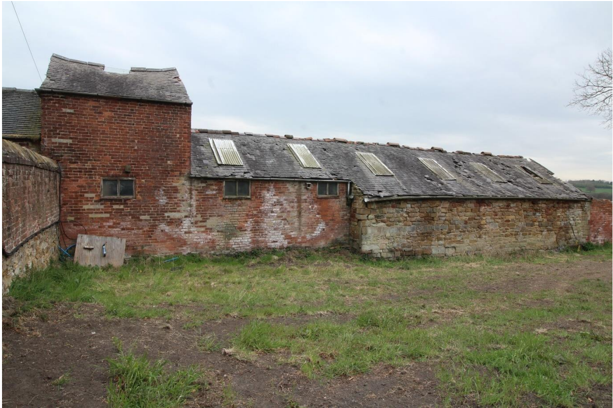
Figure 92 West elevations of Building 11 (left) and Building 4, looking east
