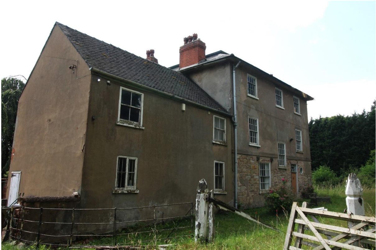
Figure 50 The east and north elevations of the farmhouse, looking south-west
