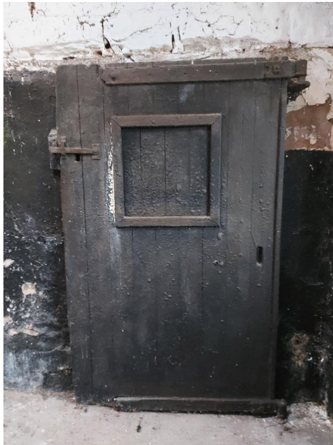
Figure 83 Door communicating between Building 8 and Building 5, looking east
