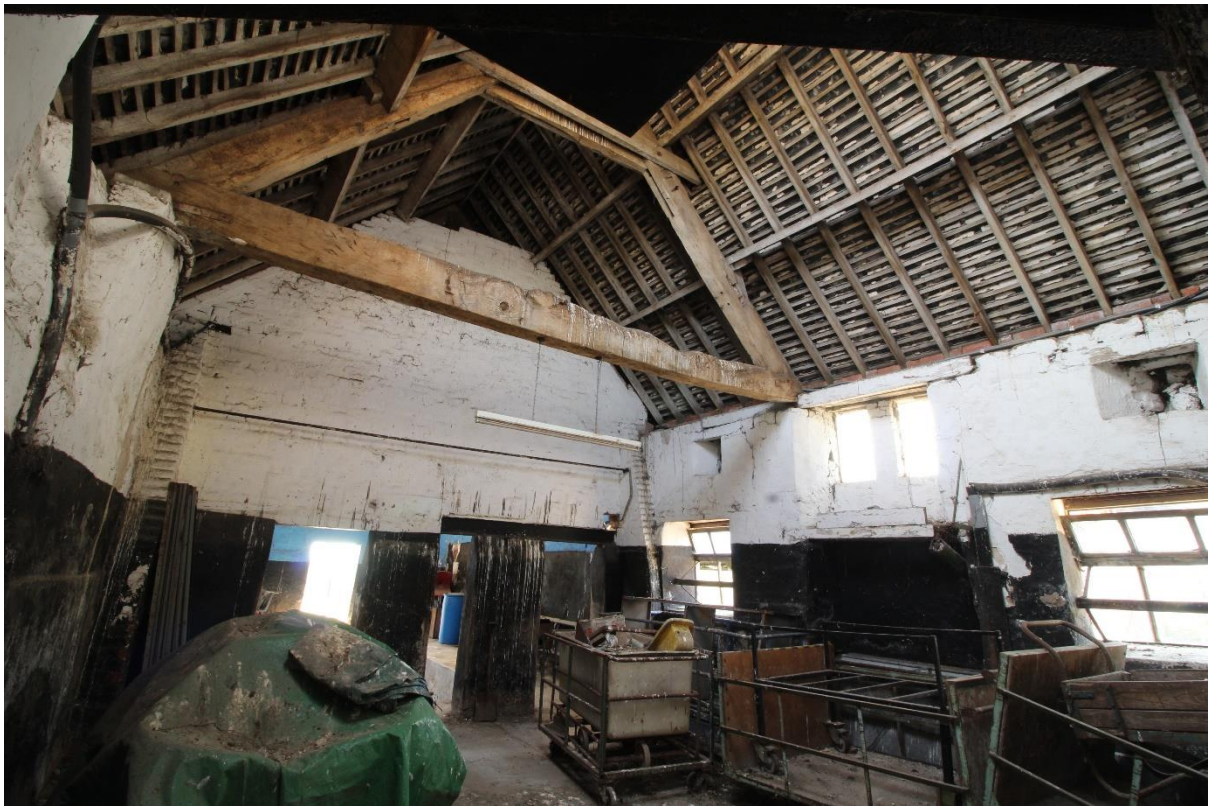
Figure 47 Interior of Building 5, looking south-west
