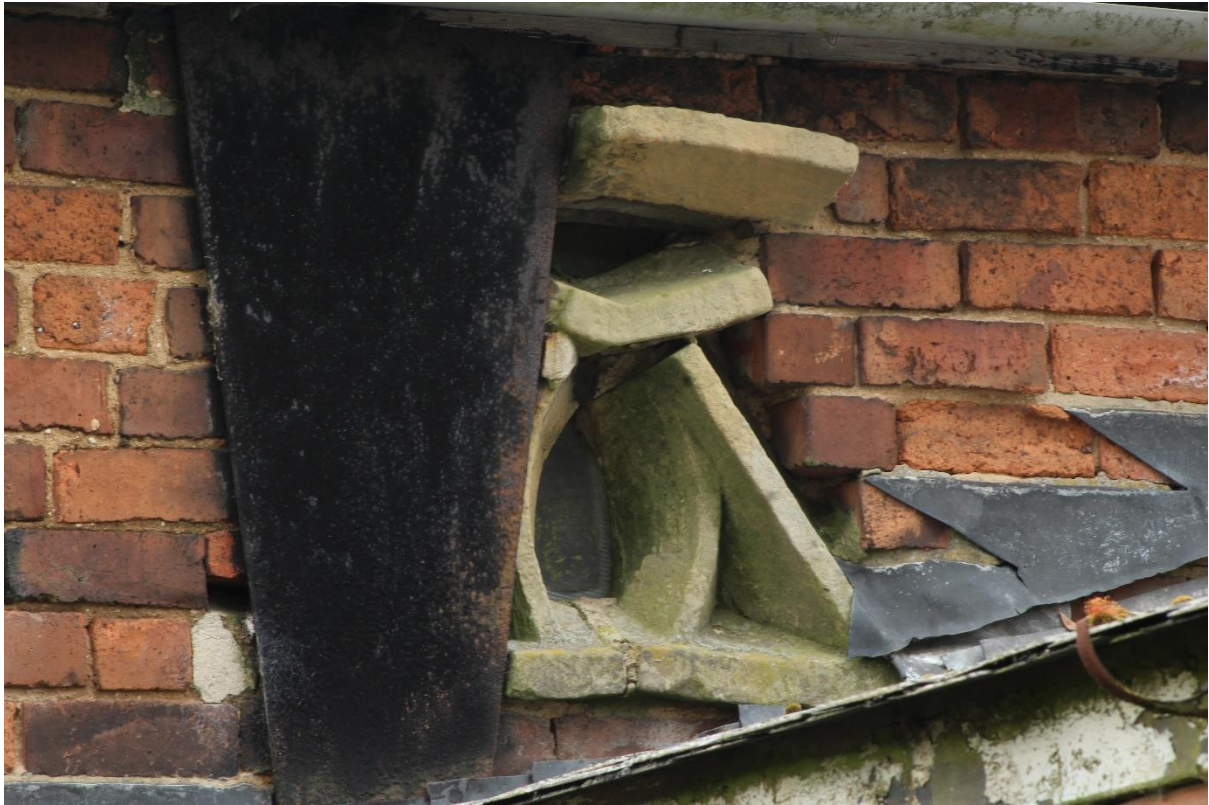
Figure 28 Four fragments of window tracery reused in Building 9 (Ex Situ Feature Number 004), looking east
