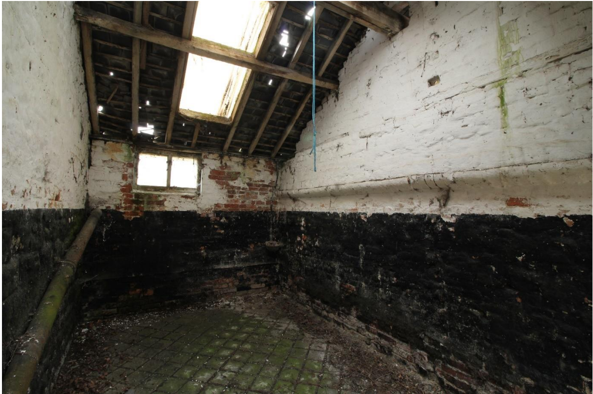
Figure 94 South bay of Building 11, looking west
