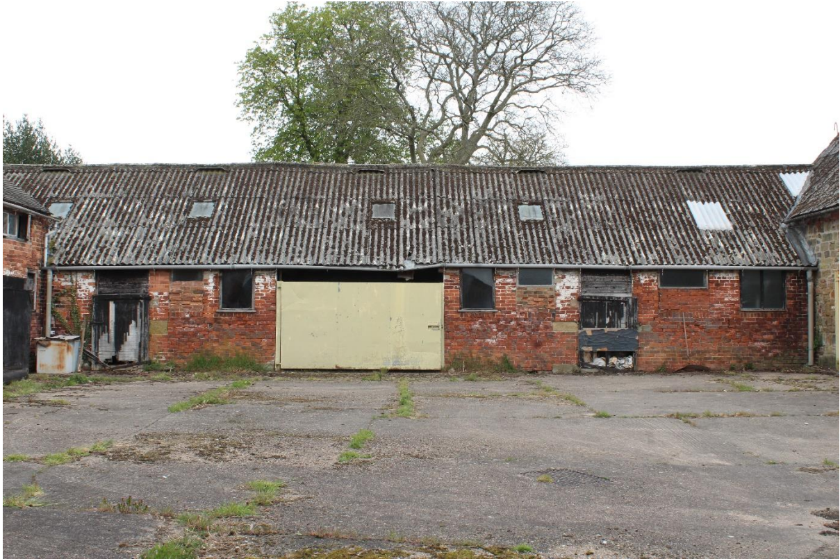
Figure 84 South elevation of Building 8, looking north
