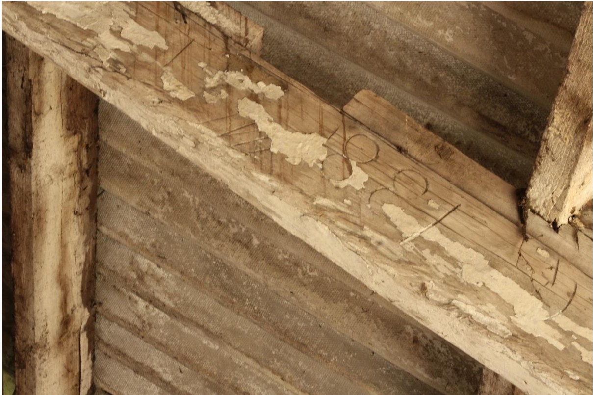
Figure 86 Baltic merchant's marks on a roof truss in Building 8, looking east
