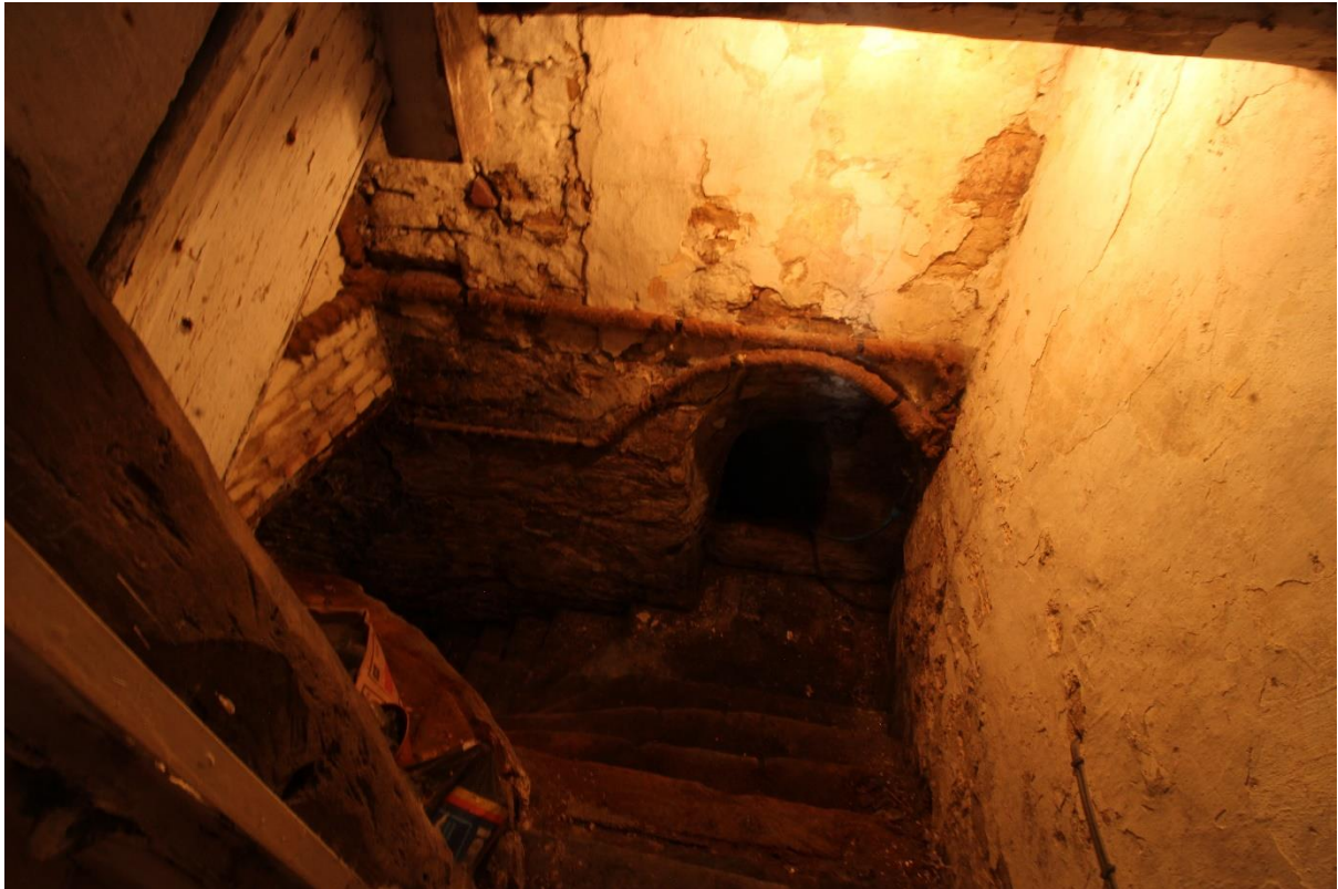
Figure 56 Stairs to the cellars, looking north
