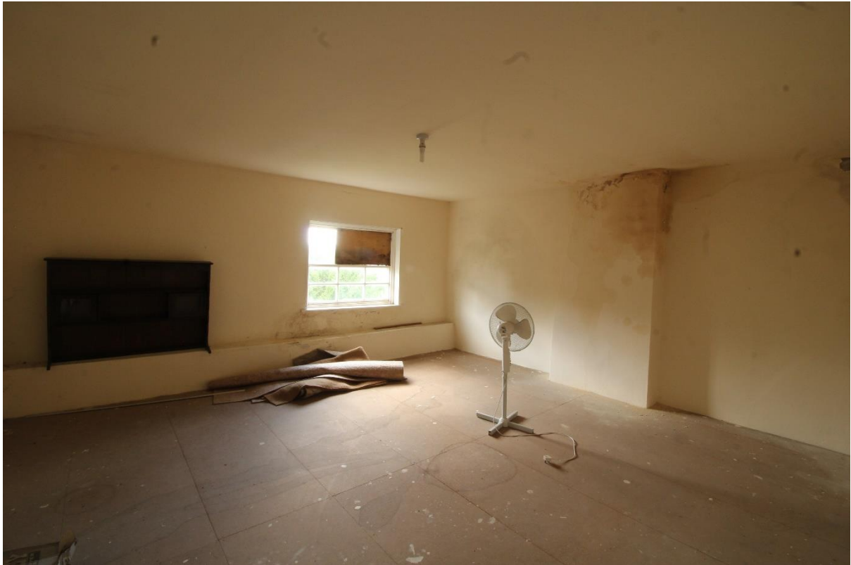
Figure 78 Farmhouse second floor south-western bedroom, looking south-west
