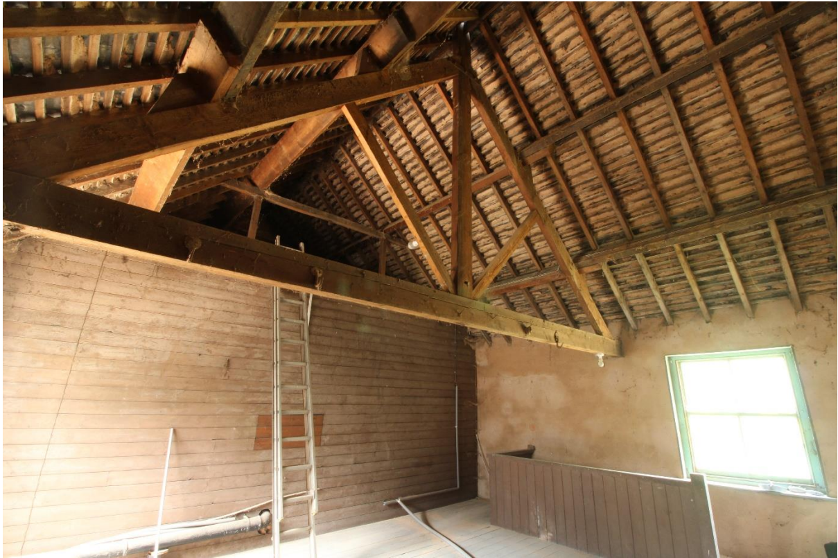
Figure 74 First floor of the eastern extension to the farmhouse, looking north-west
