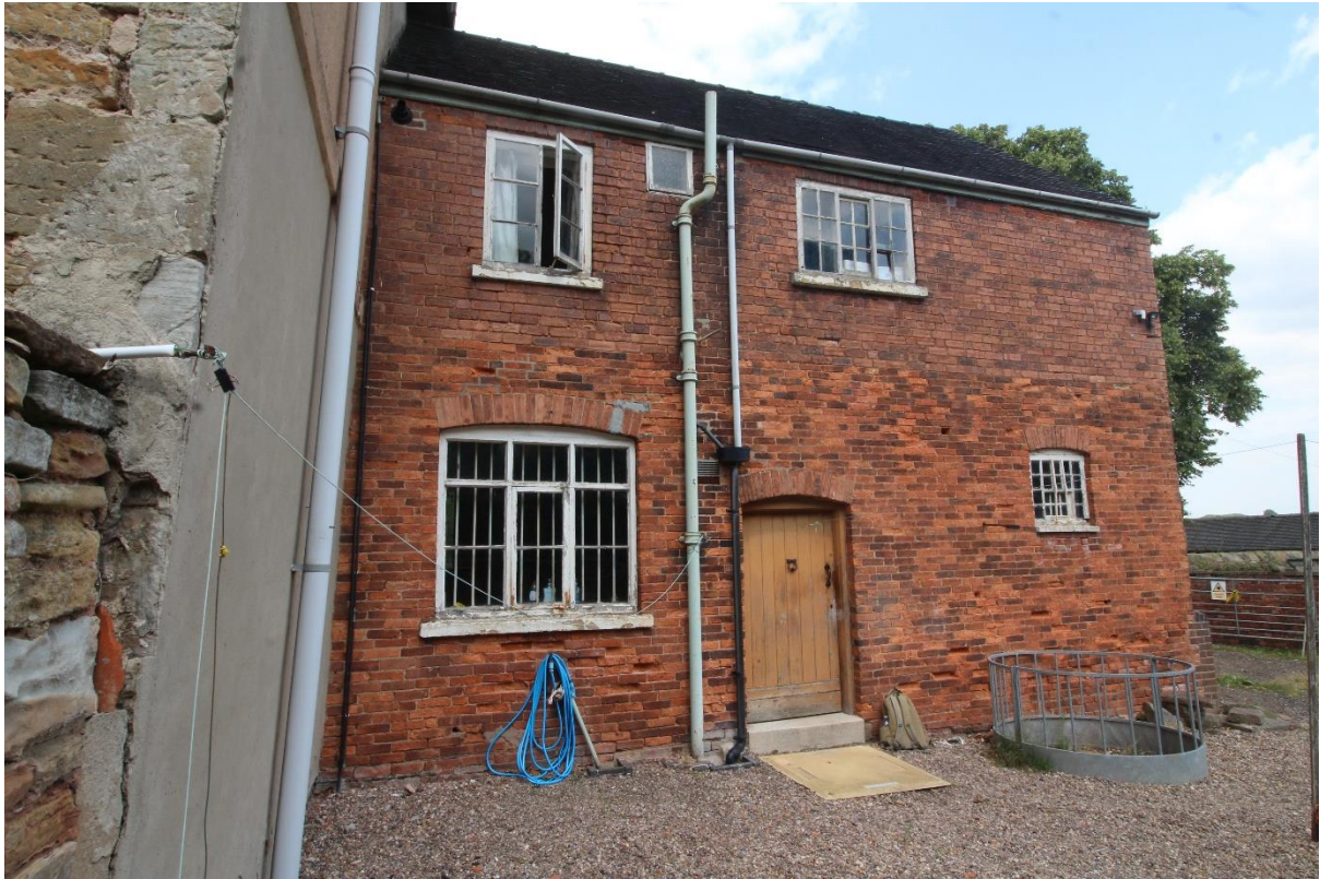
Figure 54 South elevation of the east extension to the farmhouse, looking north-east
