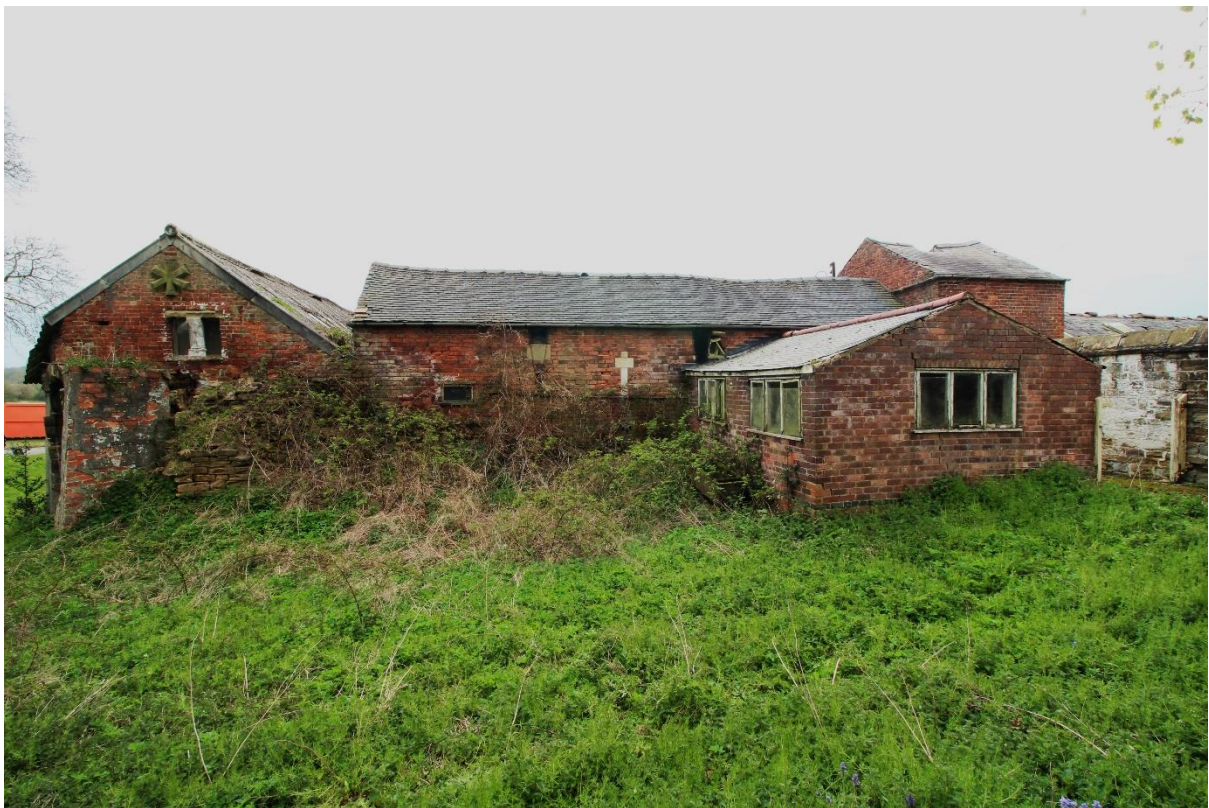
Figure 87 Exterior of the west elevations of Building 8 (right), Building 9 (centre) and Building 10 (projecting into mid-ground), looking east
