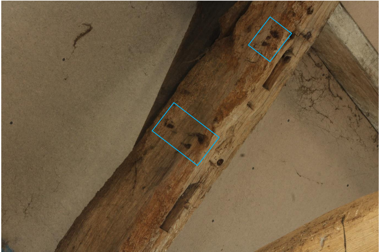
Figure 36 Possible apotropaic burn marks (outlined in blue) on north face of west rafter of Principal Truss 1, Building 5 (Ex Situ Feature Number 011), looking north-west
