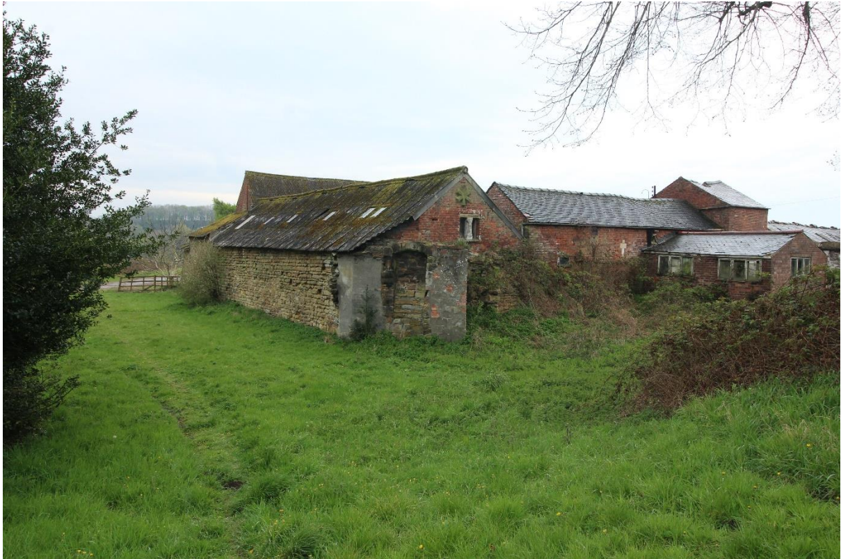
Figure 13 North-west angle of Greasley Castle, looking south-east
