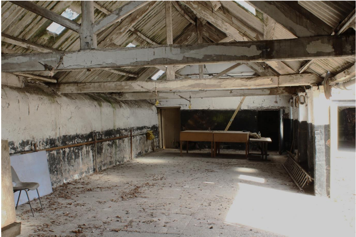
Figure 46 Interior of Building 8, looking east
