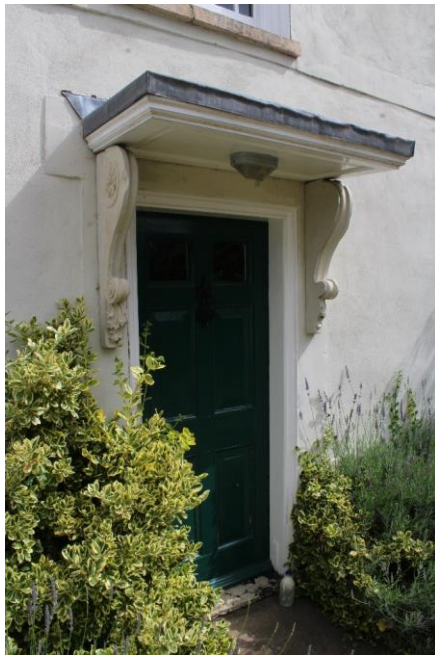
Figure 23 Porch of 12 Bell Lane. Looking north-east.
