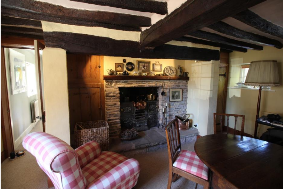
Figure 33 Inglenook fireplace in the living room of 6 Westfield Lane. Looking west. Note the spine beam.
