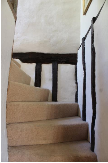
Figure 32 Staircase of 6 Westfield Lane. Looking east.
