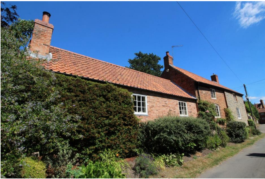
Figure 44 6 Westfield Lane. Looking east.
