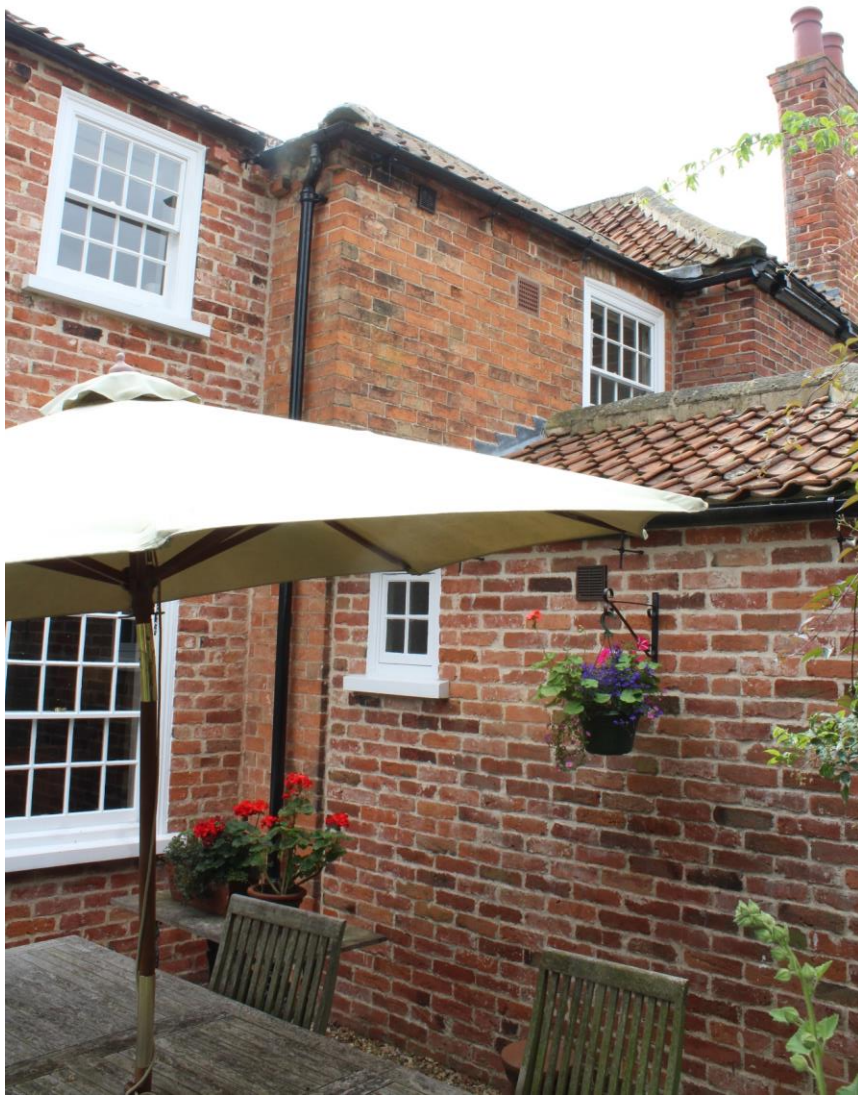
Figure 26. West elevation of 12 Bell Lane. Looking south-east.
