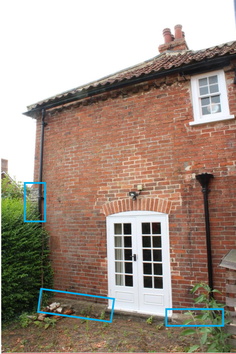
Figure 17 North elevation of 12 Bell Lane. Looking south. Note the presence of blue Lias stonework (highlighted in blue).
