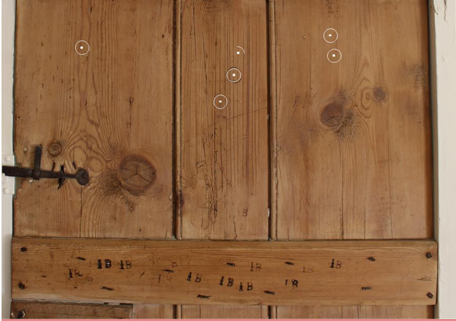
Figure 42. Scribed circles on the inner face of the door between the stair and western bedroom at 6 Westfield Lane. Looking east. Photograph has been interpreted with over-drawing.
