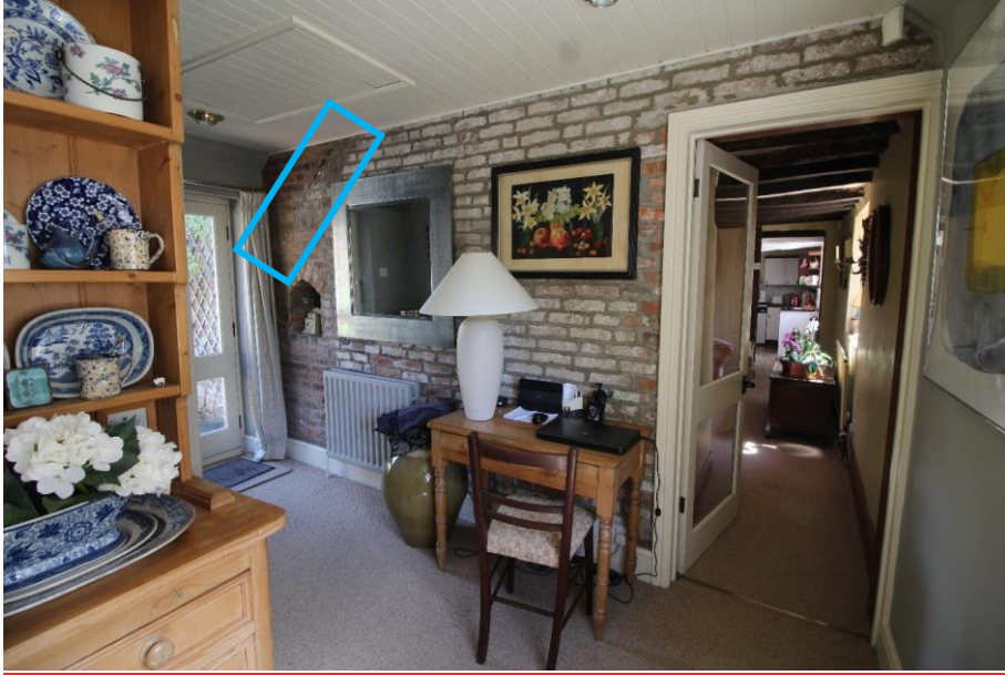
Figure 45 West elevation of the living room at 6 Westfield Lane. Looking east. Note the roof scar highlighted in blue.
