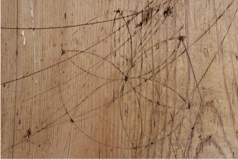
Figure 43 Scribed rosette on the inner face of the door between the stair and western bedroom at 6 Westfield Lane. Looking east.
