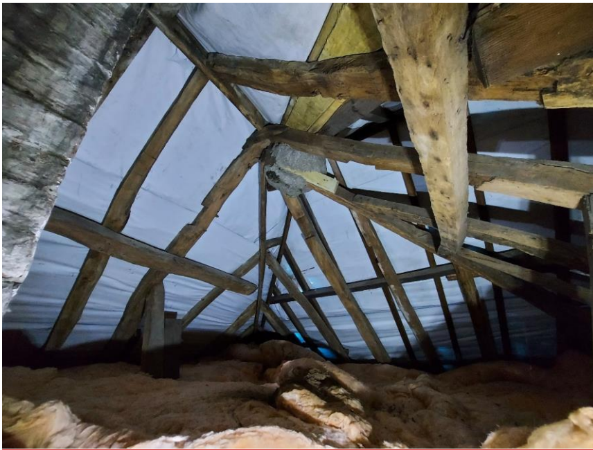
Figure 12 Attic of 12 Bell Lane. Looking south-east.
