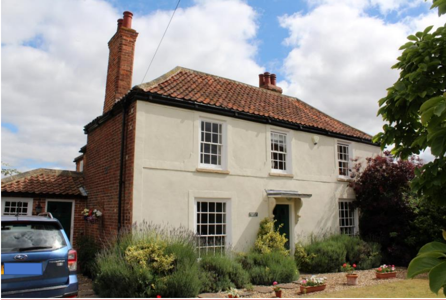
Figure 9 12 Bell Lane. Looking north-east.
