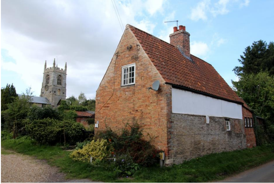
Figure 22 7 Westfield Lane, Collingham. Looking south-west. Note the blue Lias to first floor height on the north elevation.
