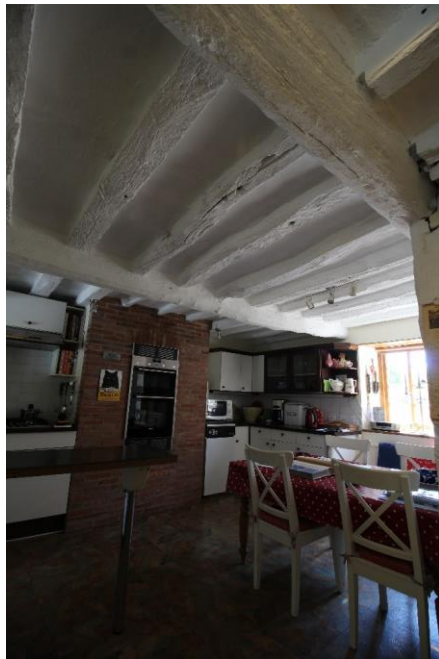
Figure 34 Kitchen of 6 Westfield Lane. Looking south.
