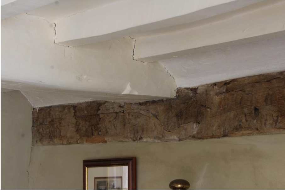
Figure 20 Detail of the spine beam of the south-eastern bedroom at the first floor of 12 Bell Lane. Looking north-east. Note the chamfer stop.
